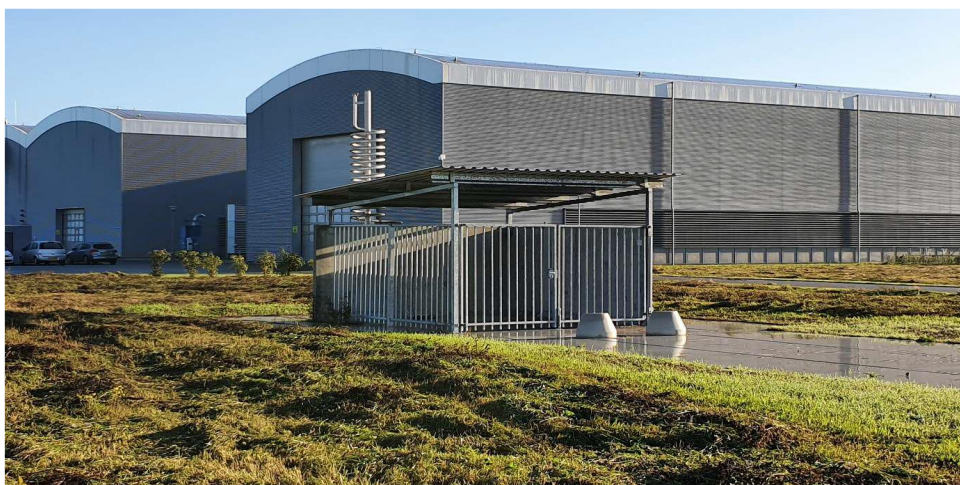
Figure 6 LH2 storage facility at NLR in Marknesse, Netherlands
