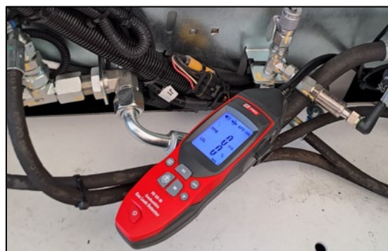
Figure 14: H2 Leakage check
