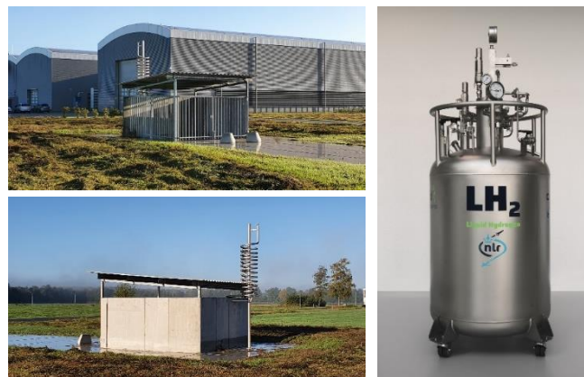
Figure 25: Example storage facility of Liquid Hydrogen at the Marknesse Facility of NLR.
