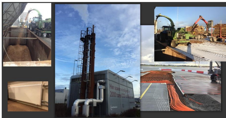
Figure 9 Biomass-fired district heating. Source: Avinor.
