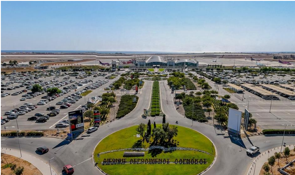
Figure 1: Larnaca Airport Aerial Photo
