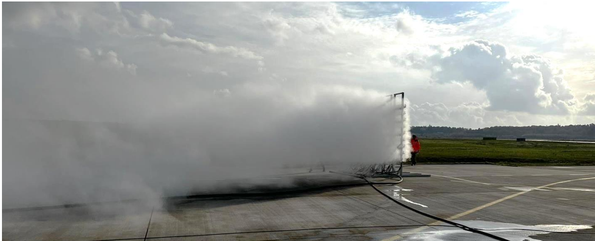
Figure 9: Picture of the water spray system operating with the flow directed into the ambient wind during pre-test 2 at EHTW.
